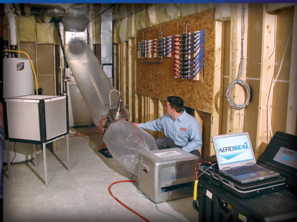
Aeroseal software allows the technician to accurately measure the duct leakage in your home
