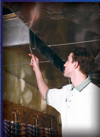
Aeroseal technician conducts initial diagnosis by analyzing airflow
