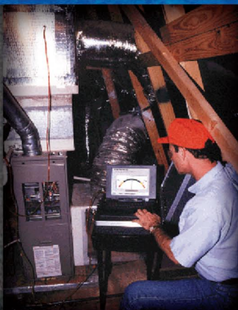
A professional Aeroseal technician will monitor the duct leakage in your home
